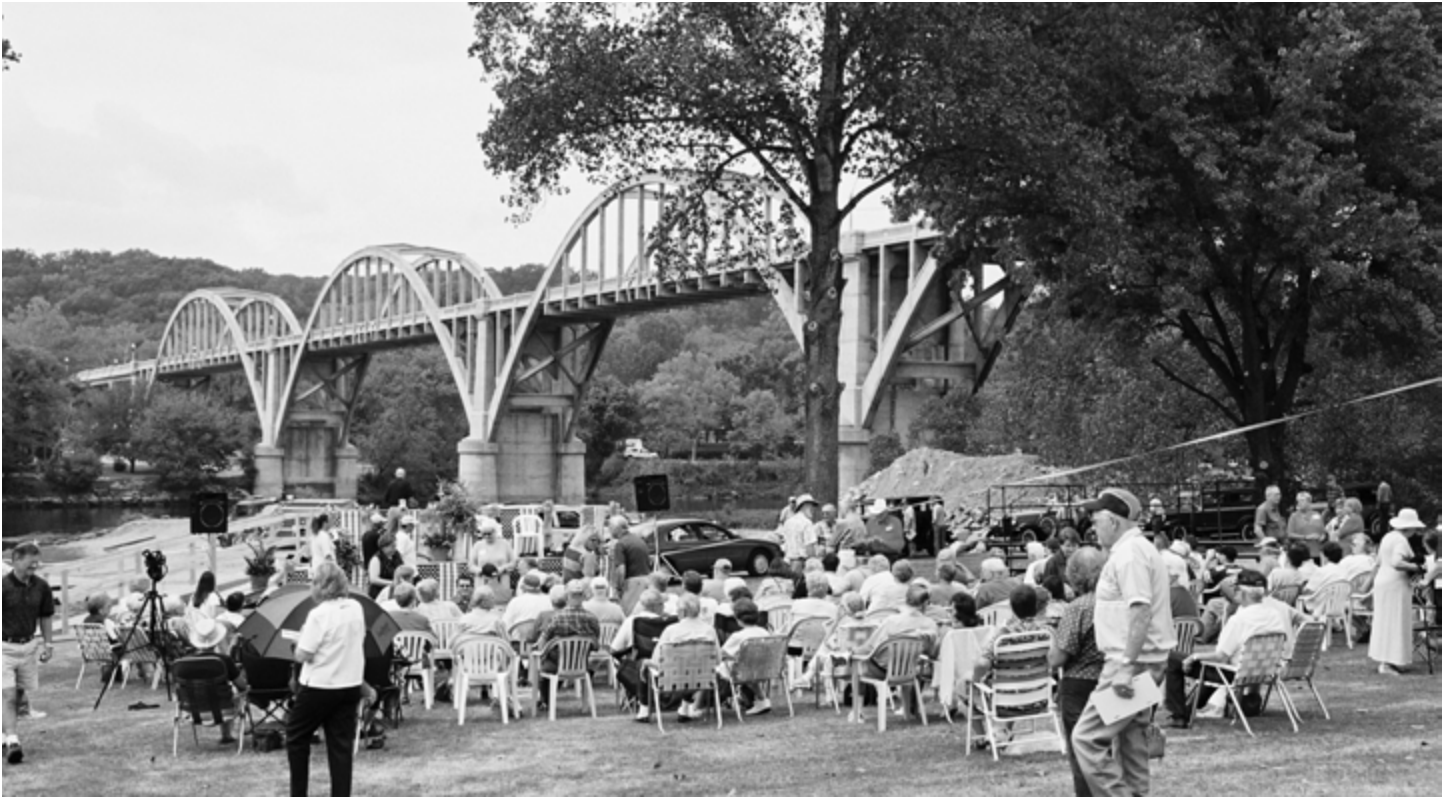
A rededication of the bridge in the fall of 2004 drew a large crowd.
