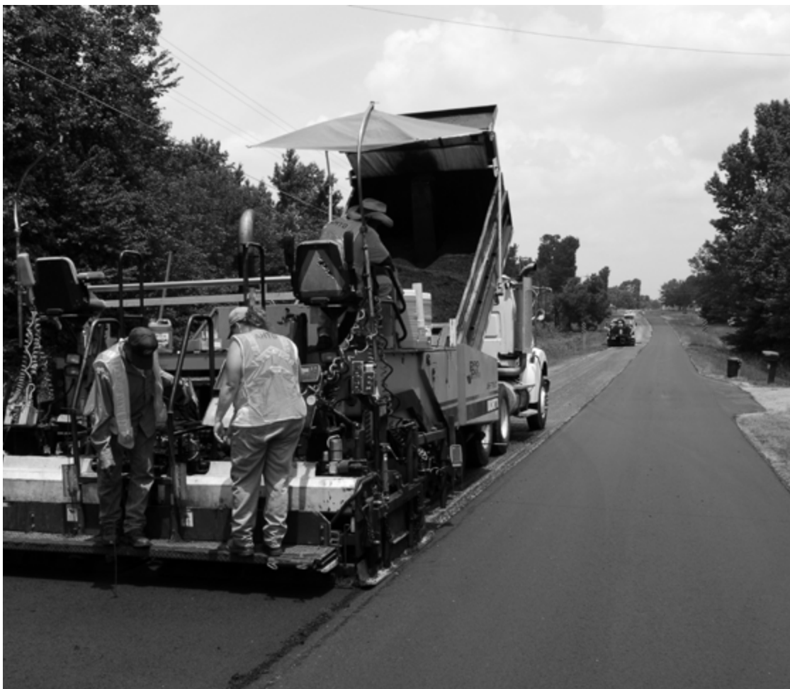
Resurfacing on Highway 321 near Cabot.
